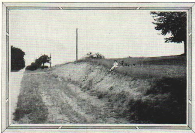
Fig. 16. Before grading. Steep roadside banks are displeasing features in informal landscape developments. (See Fig. 17.)
