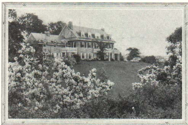
Fig. 1. The selection of a slightly spot for the house is the first important step in the development of a beautiful home grounds. 2
