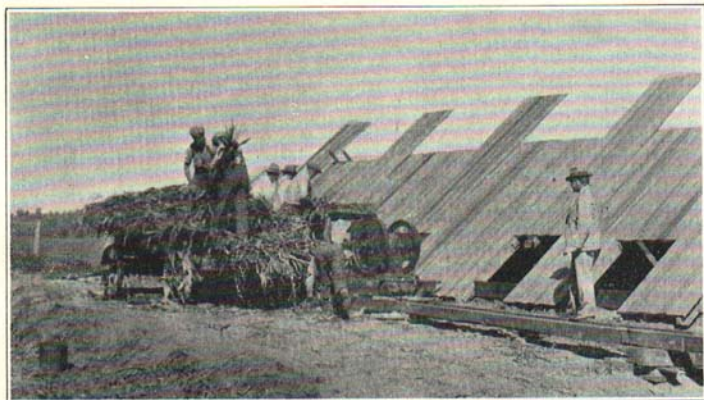
Fig. 3. Using low-cost machinery for filling.
