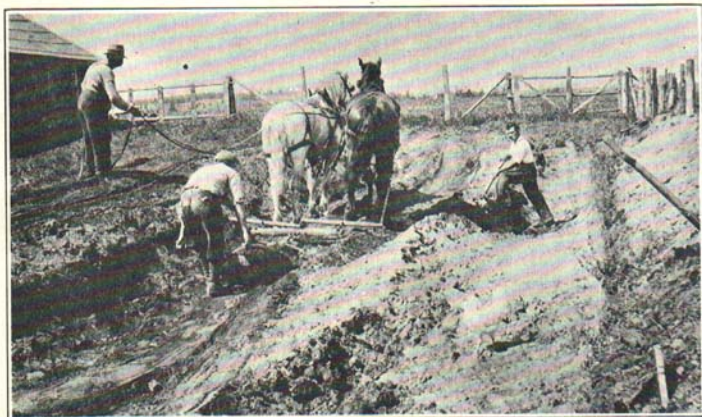
Fig. 1. Excavating for trench silo.
