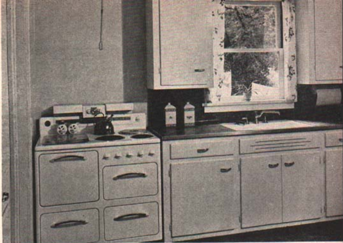
Fig. 2. One large window above the sink is usually more desirable than two small ones. This gives more wall space for upper cupboards and simplifies the curtaining problem. Notice that the faucets come out of the sink itself rather than out of a linoleum-covered surface.
