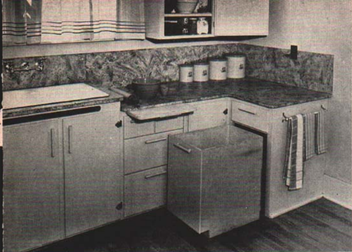
Fig. 6. A mixing cupboard in which a lower work-height has been used. Notice how the bin wastes no space, because it is flat and box-like at the bottom. It does not need to be supported when open, and it won't bang shut. The large rubber, ball-bearing casters make it easily moved. This is a larger bin than many families need. It is 23 inches deep by 15 inches wide, and will hold 100 pounds of flour or sugar. The space at the end of the cupboard has been left for a refrigerator.
