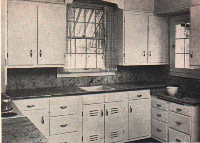
Fig. 24. An "unbroken" U-arrangement, in which the refrigerator and mixing cupboard are located at the right of the sink; and dish cupboard, range, and serving space at the left of sink. The change in work-heights has been made at the corner. Other views of this kitchen are shown in Figs. 5 and 19. (The sink is only a temporary one.) Notice slots in doors of cupboard below sink which provide for ventilation.
