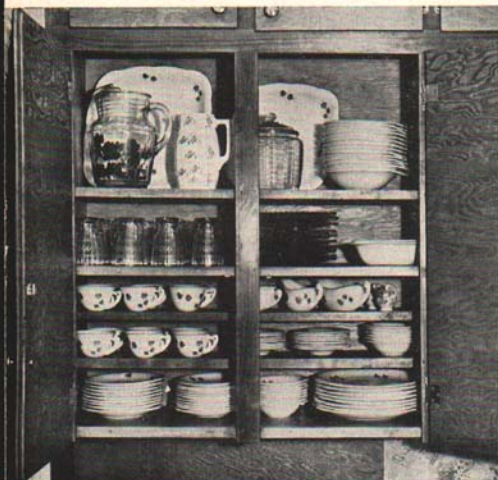
Fig. 17. There is no waste space in this dish cupboard. Only dishes of the same size and kind are stacked together. One-to-two inches of clearance has been allowed, so that the dishes can be placed on the shelf or removed easily. Cups, saucers and similar china are stored on the narrow or "half" shelves.
