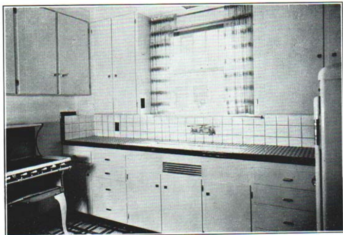
Fig. 21. A compact convenient kitchen arrangement. Notice these features: light in ceiling above sink, wall outlets for small electrical equipment, cupboards on wall space over the range, glazed tile working surface, double sink, ventilated cupboard below sink, and toe space at bottom of cupboard.
