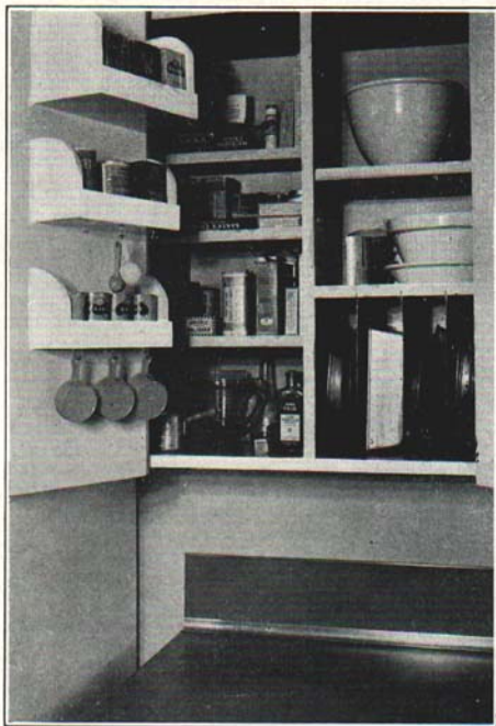
Fig. 3. This cupboard is placed next to the refrigerator and a few steps from the sink. The doors are hinged so that the entire cupboard opens wide and everything is accessible. Here are stored the staple foods and equipment necessary when such foods as a cake or biscuits are to be mixed. Notice the pockets on the door (graduated in size) where spices are stored and the vertical shelves for storing the pie and cake pans.
