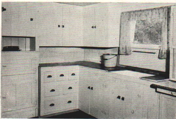
Fig. 9. A convenient food preparation and dishwashing center combination. To decrease building costs the old kitchen cabinet was placed at the right of the sink and is used as the mixing cupboard.
