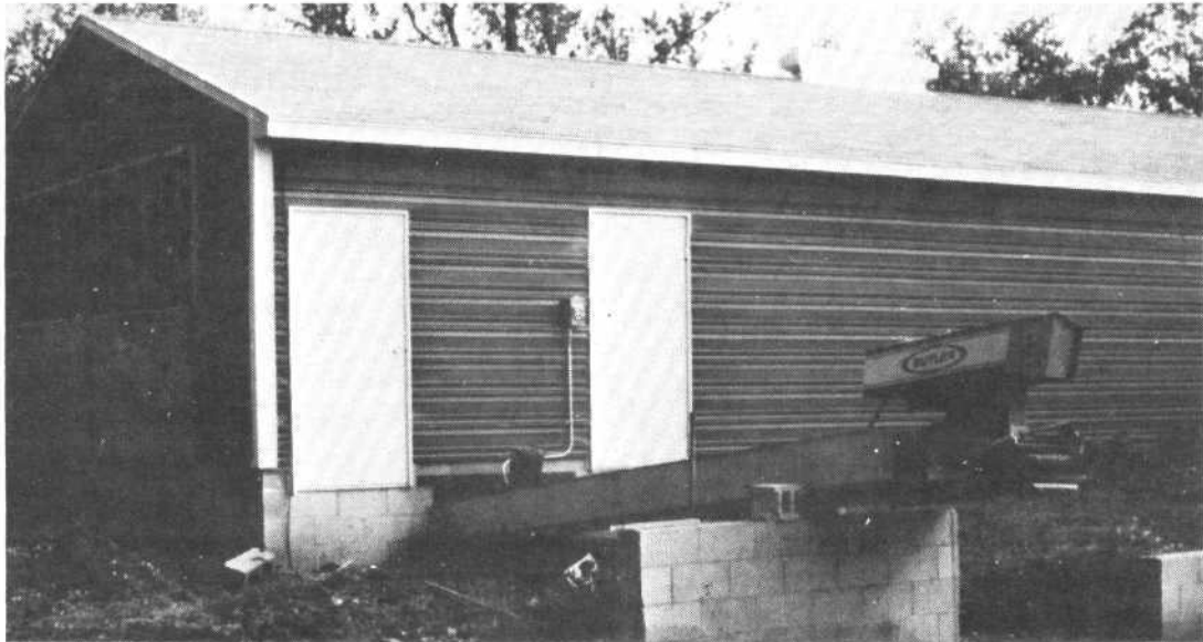
Figure 6. Traditional gutter cleaners work well in a solid manure system.
