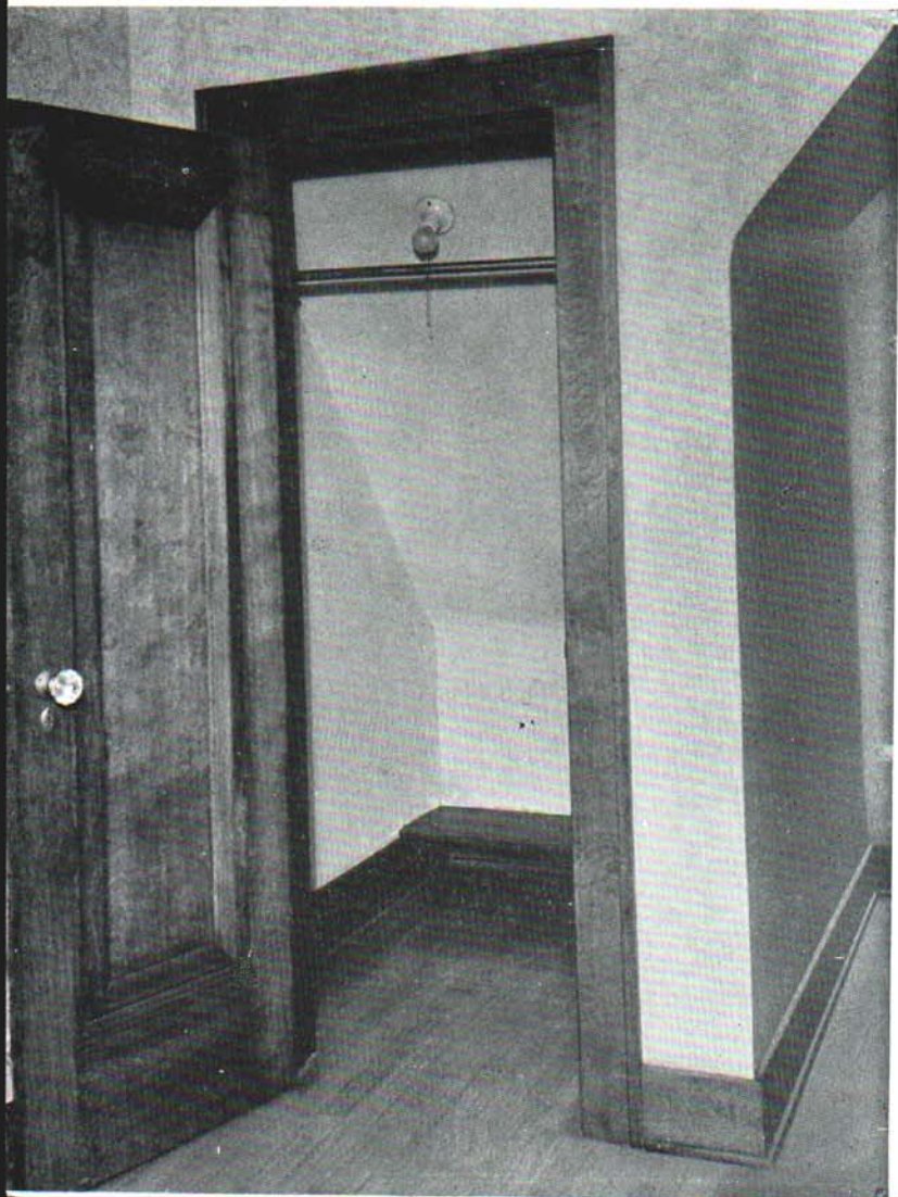
Fig. 11. Closet built under the caves.
