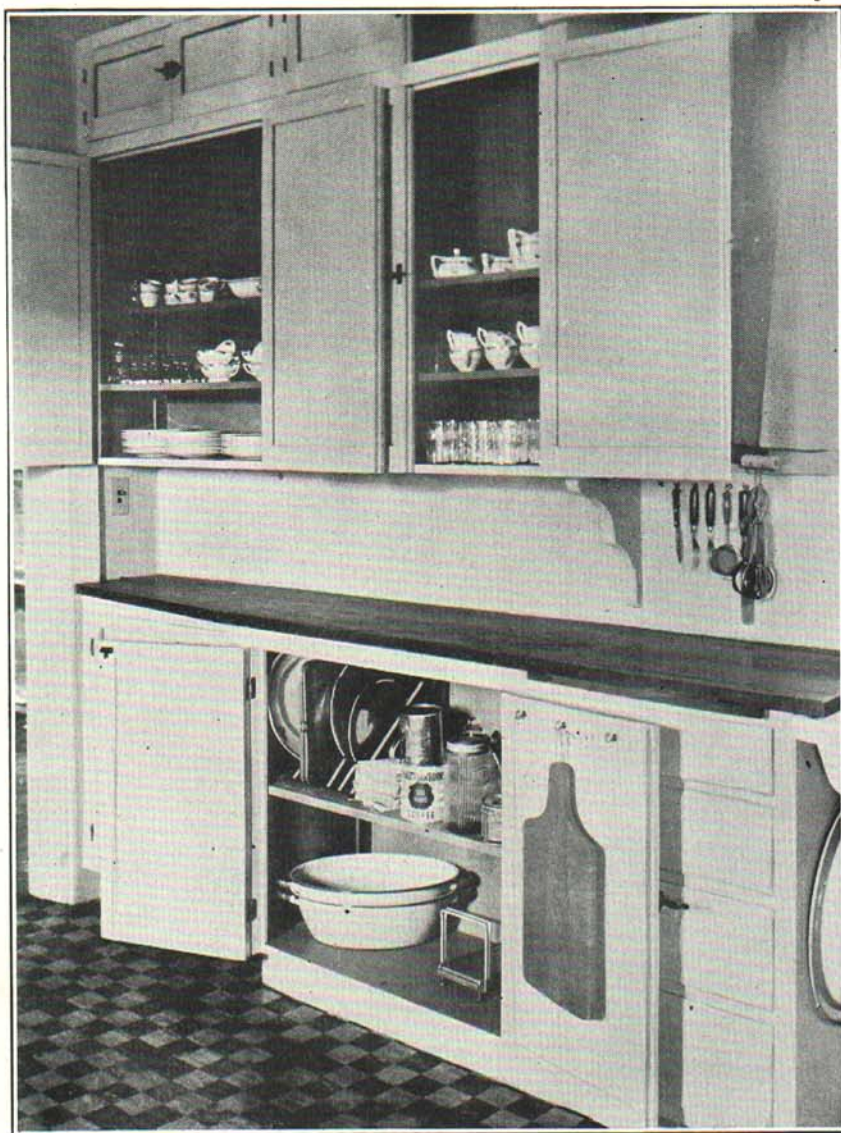
Fig. 17. A kitchen cabinet such as this one adds much to the efficiency and attractiveness of the kitchen. To increase storage space additional shelves should be added in the dish section of the cabinet. Note the rack in lower section for storing lids and pie tins in upright position. Vertical shelves might be used in place of this rack. The hooks for frequently used small articles facilitate ease in food preparation.
