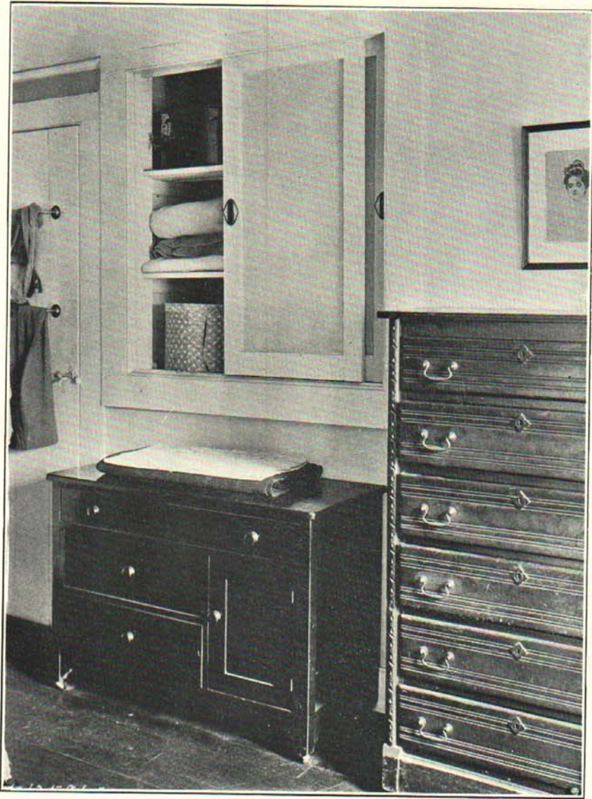
Fig. 12. A bedding and luggage cupboard which extends into the attic. Sliding doors are used to conserve room space,
