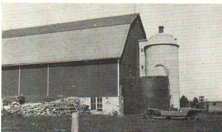
Fig. 2. A temporary crib silo beside a permanent silo. Courtesy of American Lumberman.
