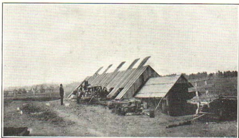
Fig. 7. A covered trench silo. The cover is constructed with alternate sections removable for convenience in filling.
