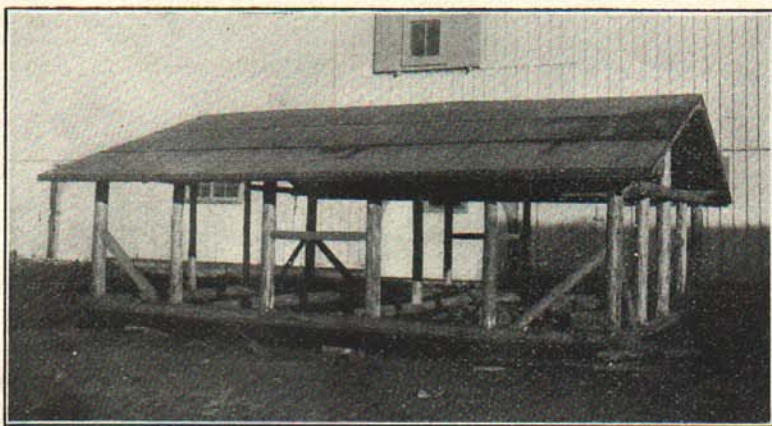
Fig. 10. Showing a summer shelter before wire netting was put on the walls. This building is 12 x 12 feet and will accommodate 100 growing turkeys.
