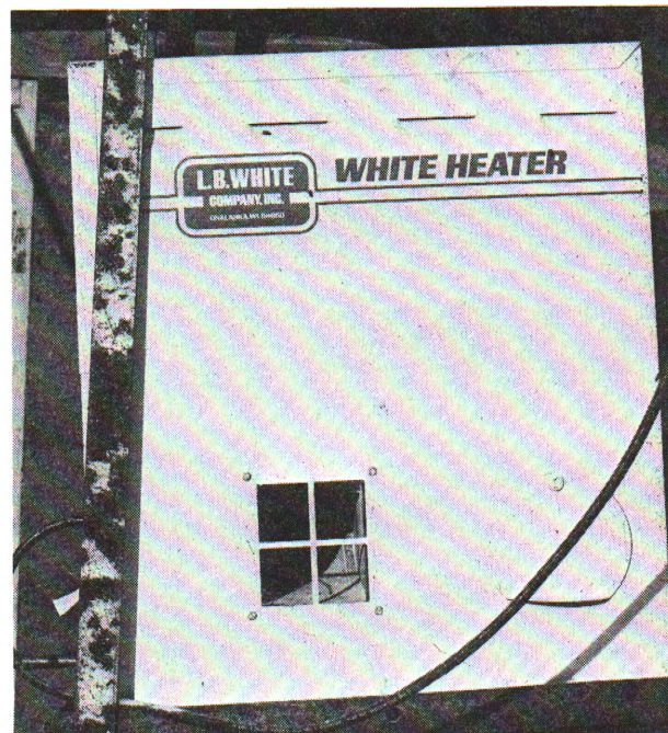
Figure 1. The discharge side of a typical centrifugal fan unit heater. Heater is hung from the ceiling and placed near an outside wall.
