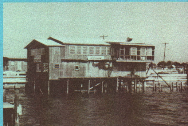
Fig. 15. (Left) Fishing piers are commonly made with salt-treated decks and creosoted or PCP-treated piling in fresh water. Fig. 16. (Right) Buildings such as this restaurant are supported on treated piles.
