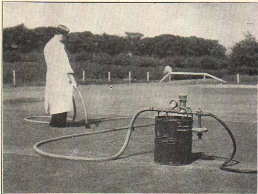
Proportioning machine in operation
