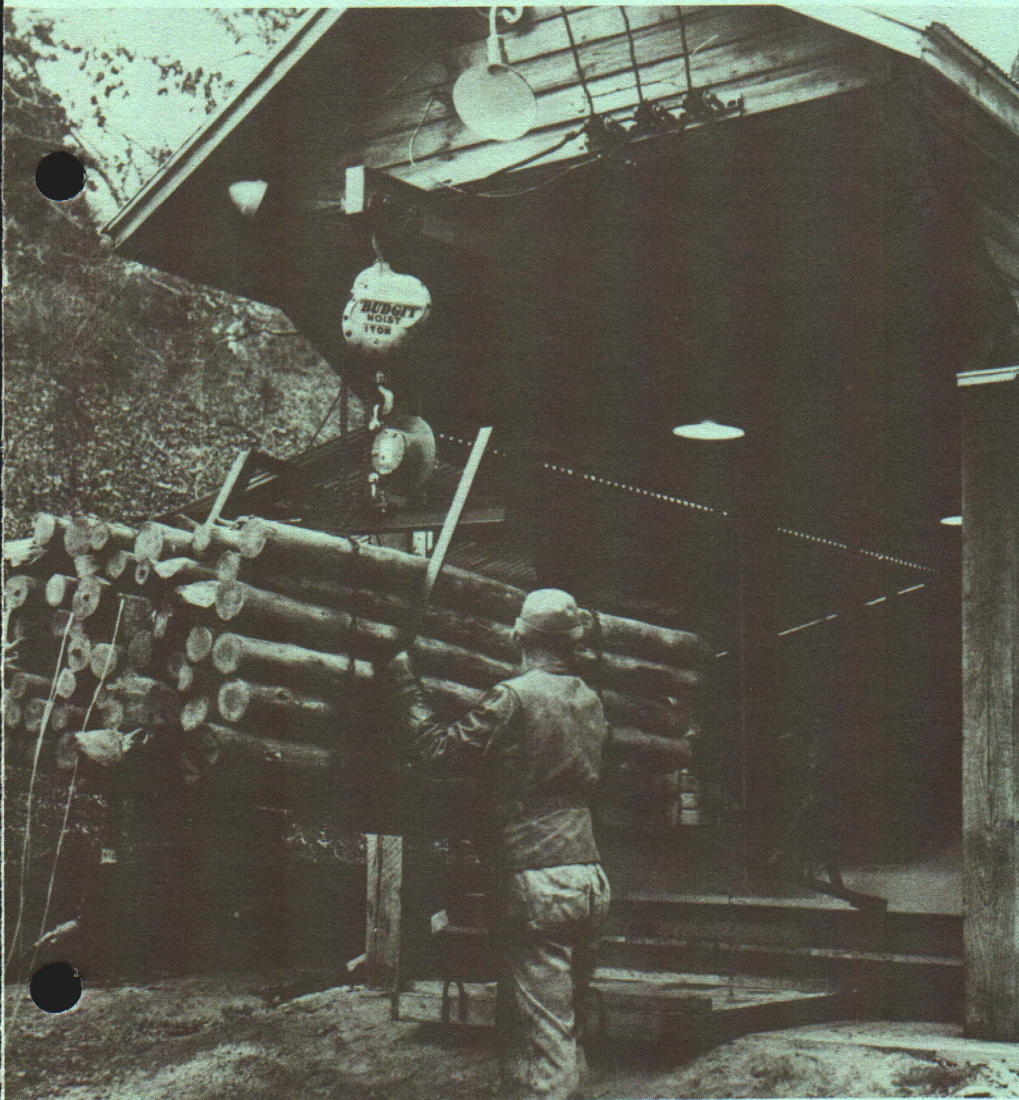
Fig. 4. (Below) Immersion treating of posts. (Photo courtesy TVA, Forestry Division.)
