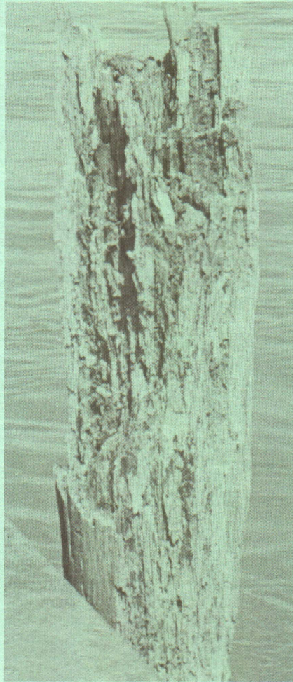
Fig. 9. (Left) Deterioration of unprotected pile. Fig. 10 (Above) Metal cap to protect piling. If metal is broken, water can enter and protection is reduced. Coal tar pitch or grease preservatives also can be used.
