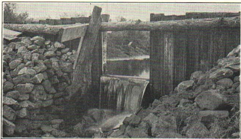
Fig. 7. The most successful grower is the one who has the water supply in his muck at his control. This picture shows one of the most efficient types of dams, constructed of interlocking sheet steel piling driven well into the muck and reinforced by rock piled on the lower side.
