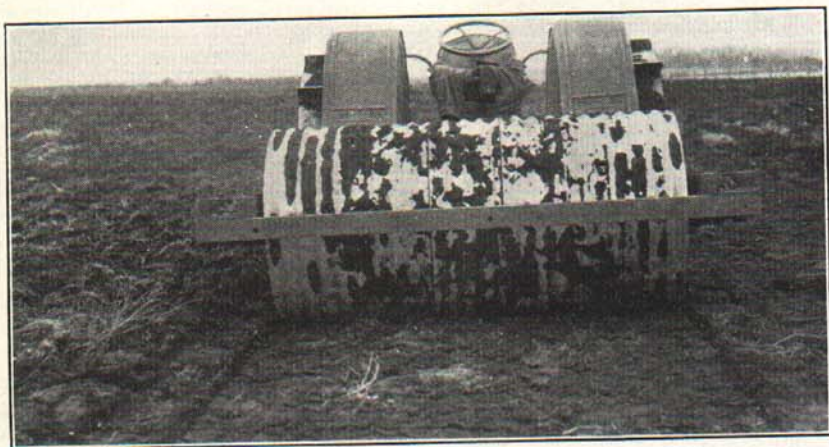
Figure 9.—The effects of the 30-inch concrete roller is evident on this rather fibrous muck. Note that the roller produces considerably more compaction than do the tractor wheels. Three or four good horses can handle a five-foot roller of this type.
