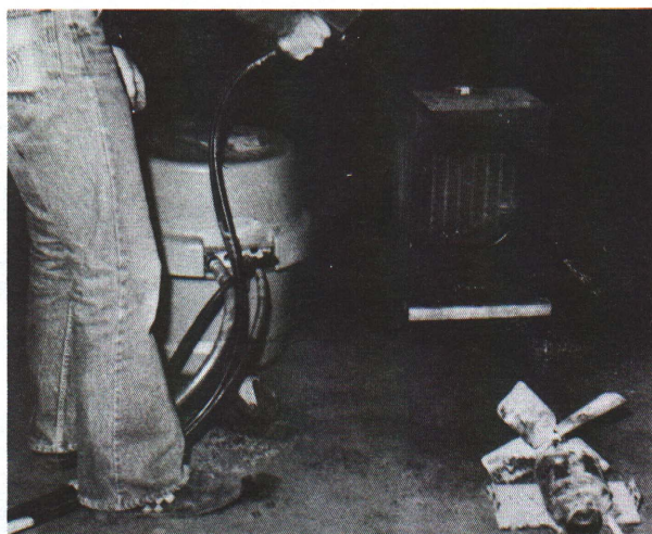
Figure 8. A pressure-washer being used to clean out the fins of an air heater. Note the fan is removed, as it has an open motor.
