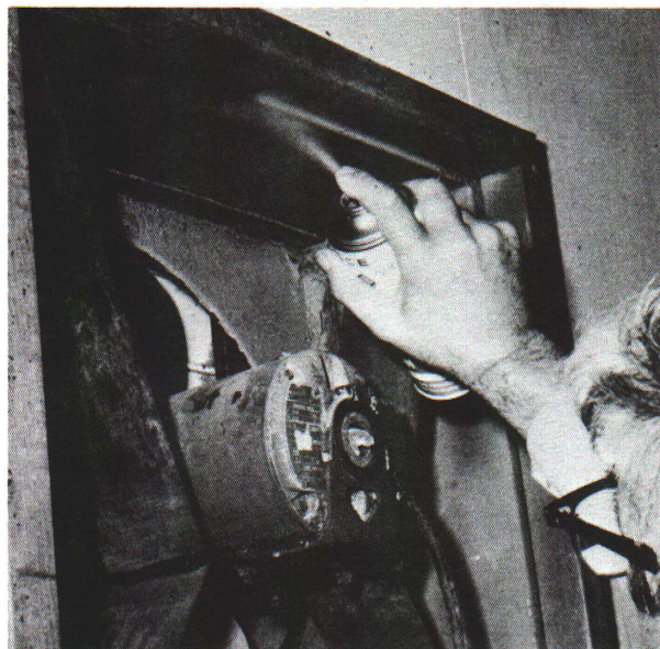
Figure 3. Repainting a fan housing after it has been cleaned and the bare spots have been primed. Keep a record card on fan maintenance near the fan.
