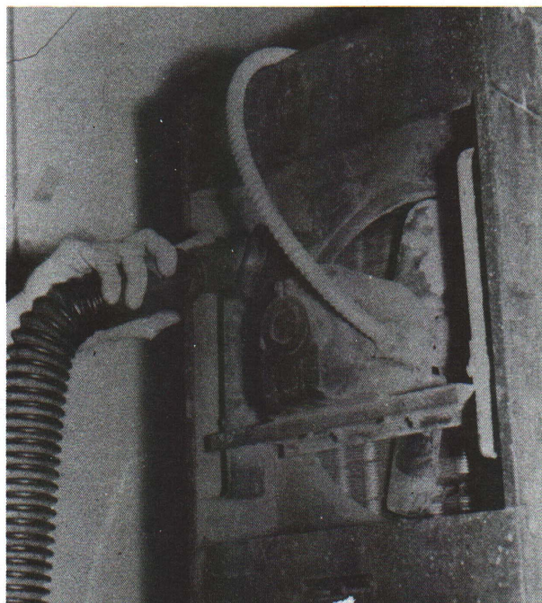
Figure 7. Use a vacuum cleaner and a stiff brush to clean off equipment.
