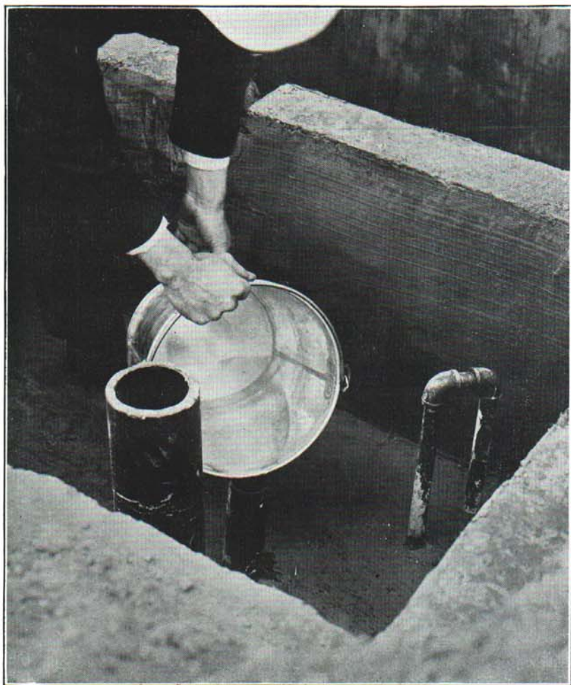
Fig. 14. Filling the siphon with water.
