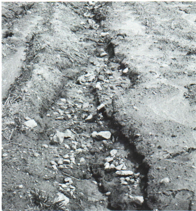
Figure 2. Rill erosion on fall-plowed hilly crop land in Ingham County.
