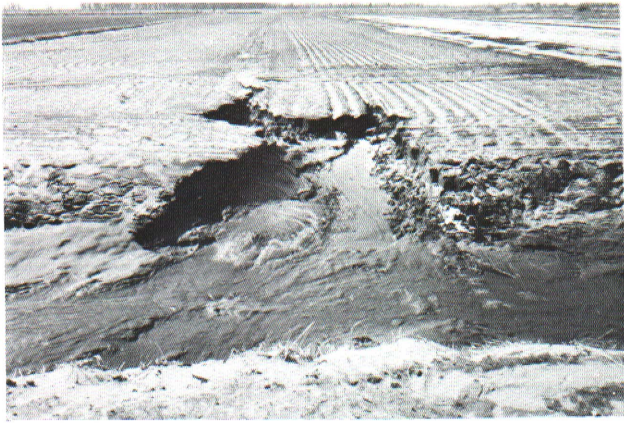
Figure 3. Shallow gully erosion on flat land in Saginaw County. Erosion is occurring where water enters road ditch. This resulted after road was improved. No vegetation was ever established on the ditch banks.
