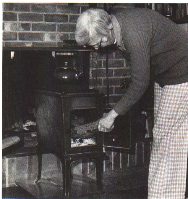
A wood stove is much more efficient than a fireplace as a source of heat. This one was installed in front of an existing fireplace.
