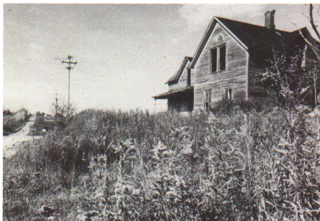
High and dry... and abandoned, when the owner found out too late that there wasn't adequate groundwater available for a well.
