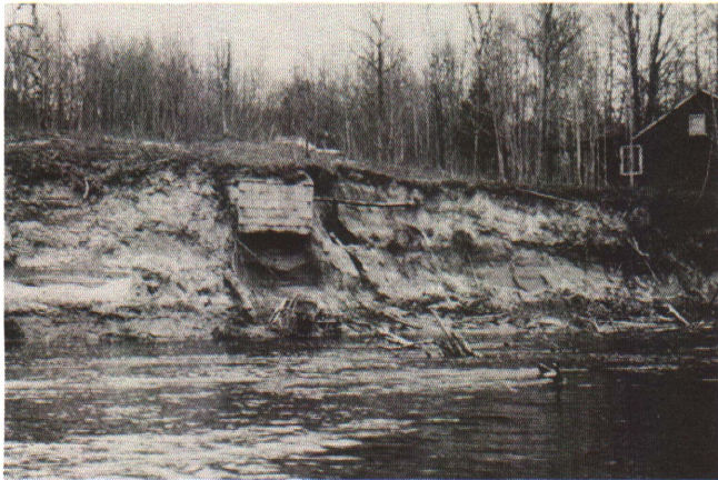
A receding bluff has left an unexpected and costly property loss: an exposed septic tank and drain field.
