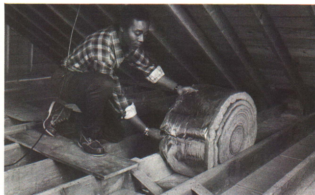
Summer cottages and most old homes need insulation in the attic or heating costs will soar.
