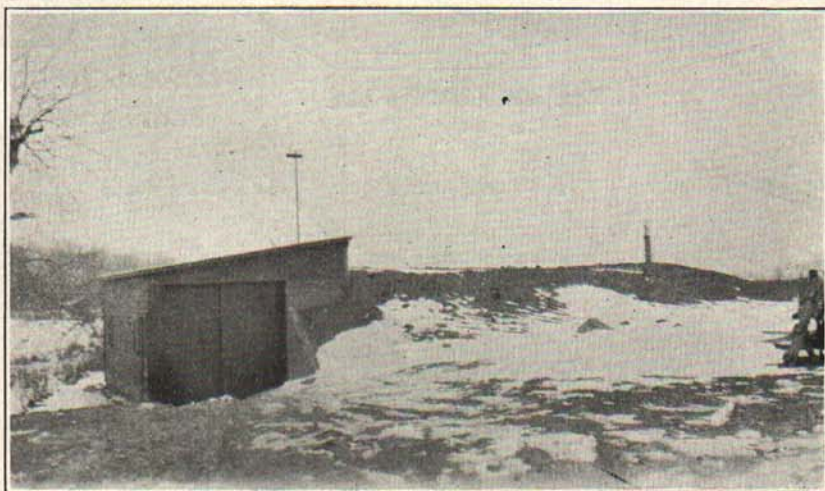
Fig. 5.—An underground cellar with driveway across one end. The small ventilating flue was found to be inadequate.
