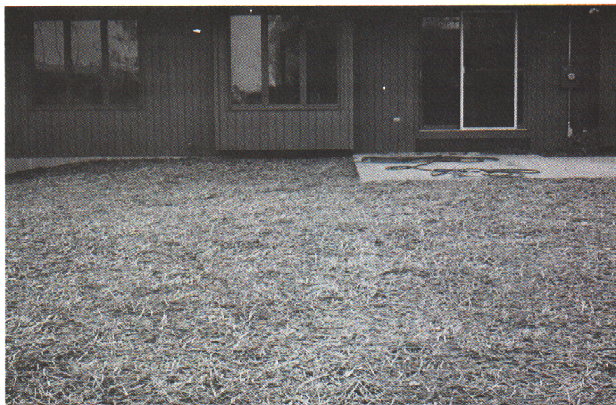
A straw mulch stabilizes the seed and soil and conserves moisture, improving germination.
