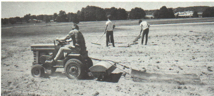
Final soil preparation requires repeated raking and leveling.
