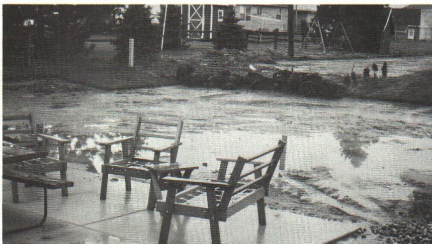
Improper grading causes water to collect on the site.
