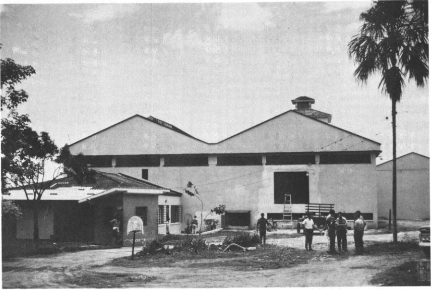
A bag storage facility for grain in Buga, operated by INAGRARIO, a public agency.
