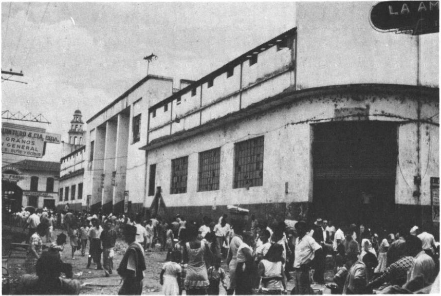
The Galeria Central building constructed in 1941 to serve as the plaza market for Cali. This facility is located in the central area of the city.
