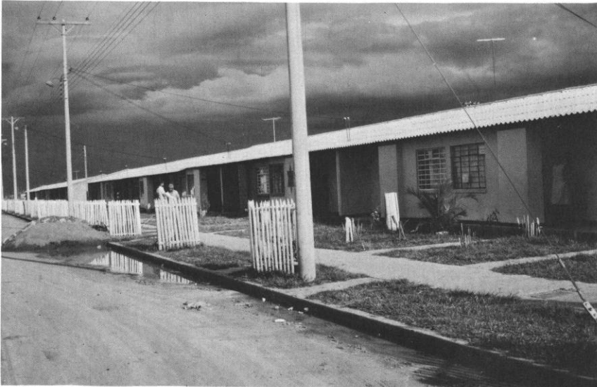
A housing project being developed by the Instituto de Credito Territorial with financial support from the Interamerican Development Bank.
