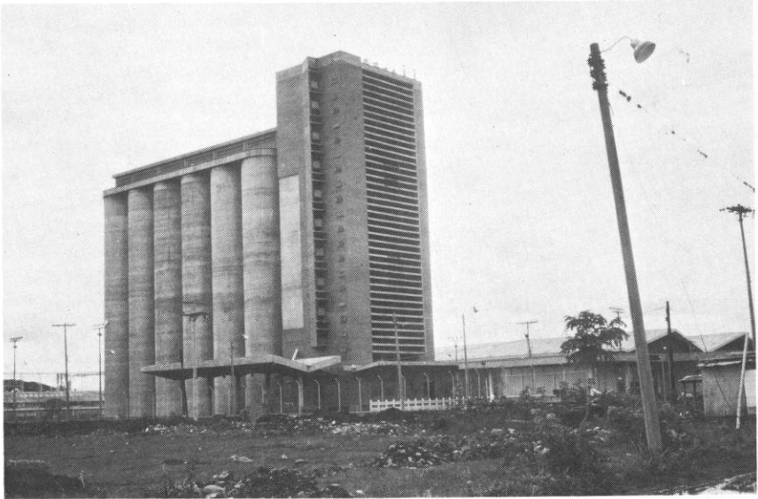
Silo grain storage facilities owned by a Colombia bank and located in Cali.
