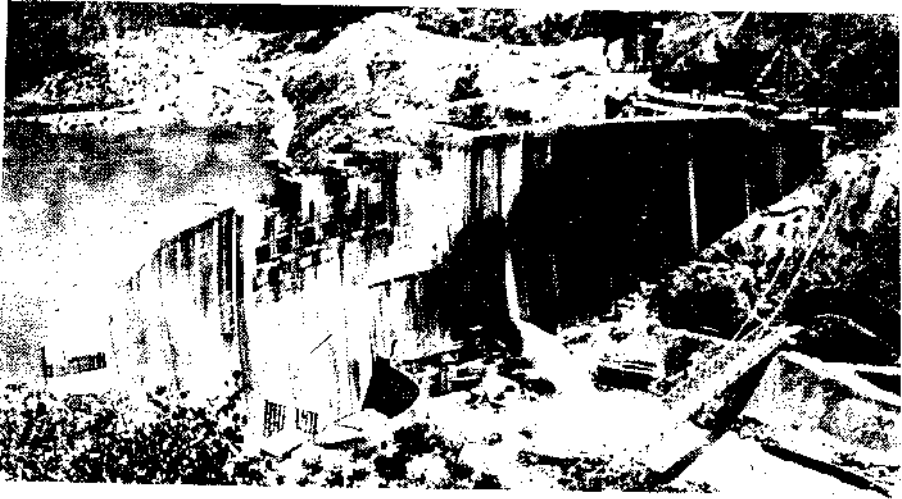
Figure 16: KARIBA DAM DURING CONSTRUCTION 1959
